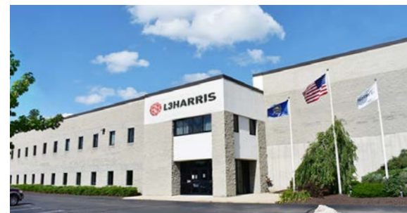
Londonderry, New Hampshire, U.S.A. facilities
